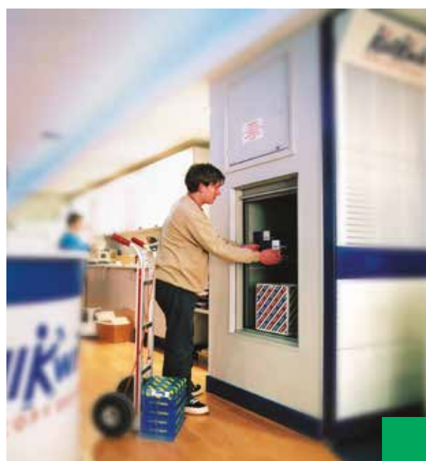
Installation in a copy centre (UK), model 100 kg, car and doors in stainless steel AISI 304.
